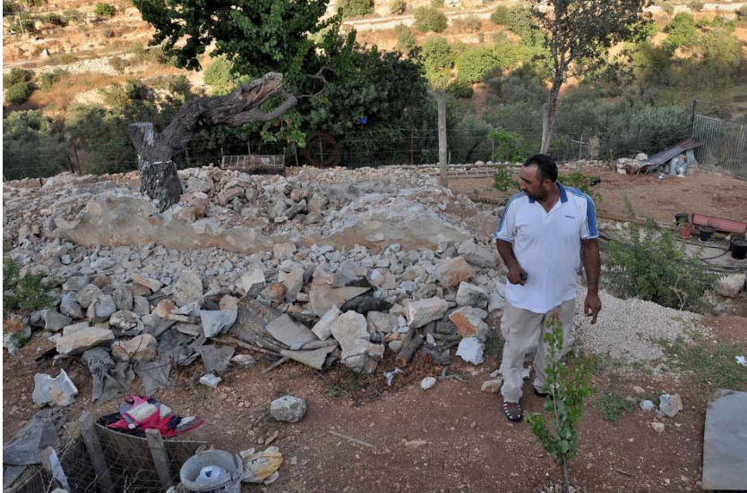
Figure 5. Tony H. standing beside his demolished farmhouse shortly after demolition. Photograph by the author.
